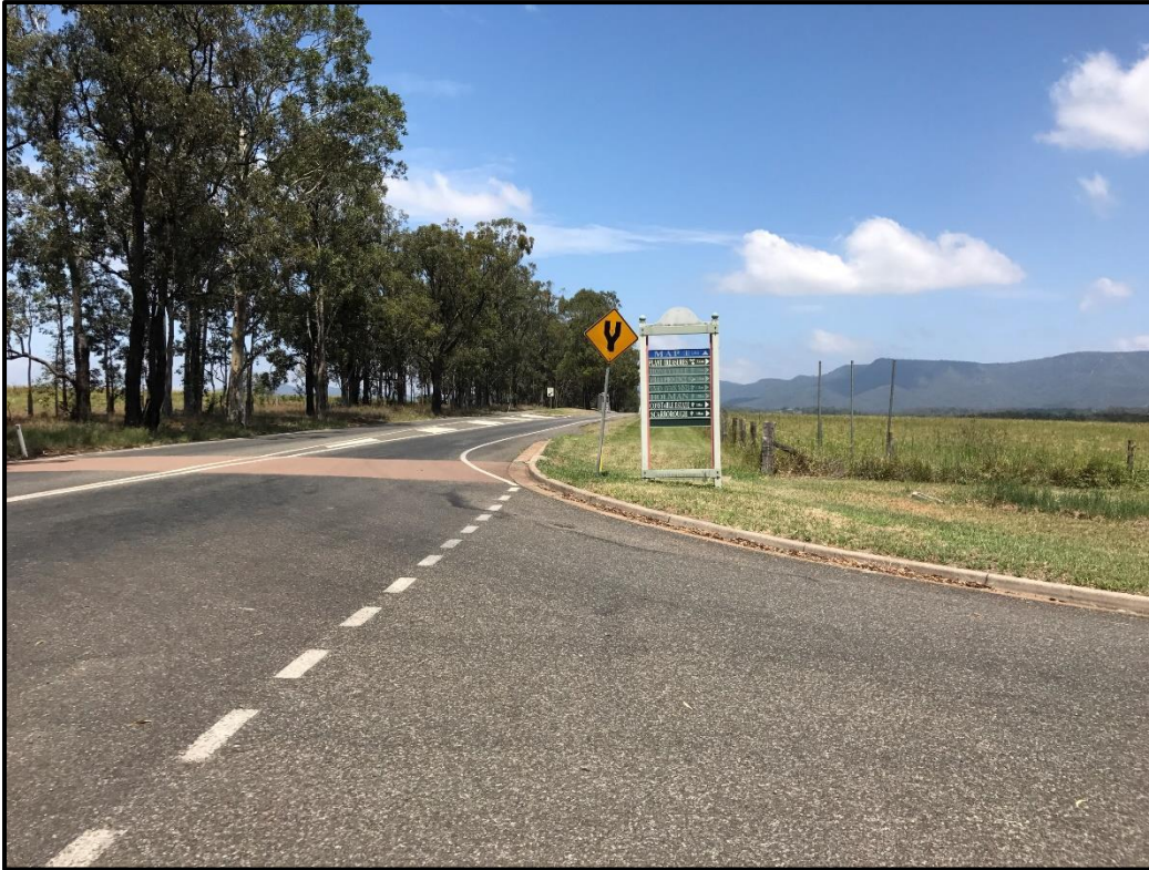
Photo 5 – Visibility looking right (south) along McDonalds Road from the intersection with Gillards Road. Shows existing tourist signage which impacts upon the sight lines for drivers turning onto McDonalds Road.
